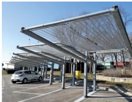
SPECIAL PRODUCT Pensiine Autogrill, Italy
